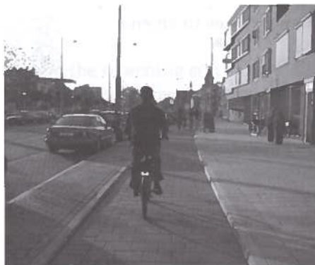
This "cycle track" in Amsterdam is on a separate level from both motorists and pedestrians.
